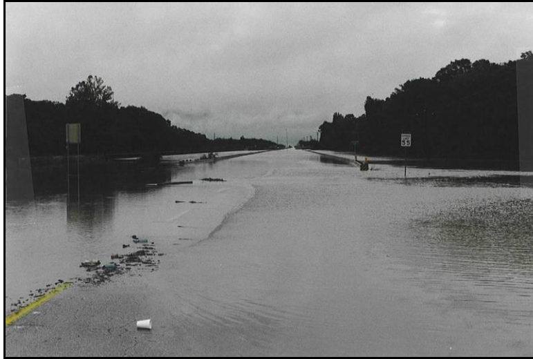
Figure 3: Floodwaters overtopping US 90A, East Bernard, TX (1998)
